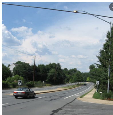
Layhill Road looking north from Bonifant Road
