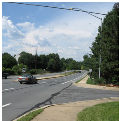
Layhill Road looking north from Norvale Road
